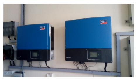
Figure 4: Existing string inverters of capacity 20 and 25 kW, connected to the 40 kWp RTPV system
