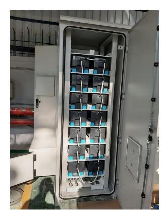
Figure 6: Snapshot of the (internal) battery bank showing 14 battery modules in series. The total energy capacity of the bank is 43.5 kWh. Specifications of the entire battery bank:
